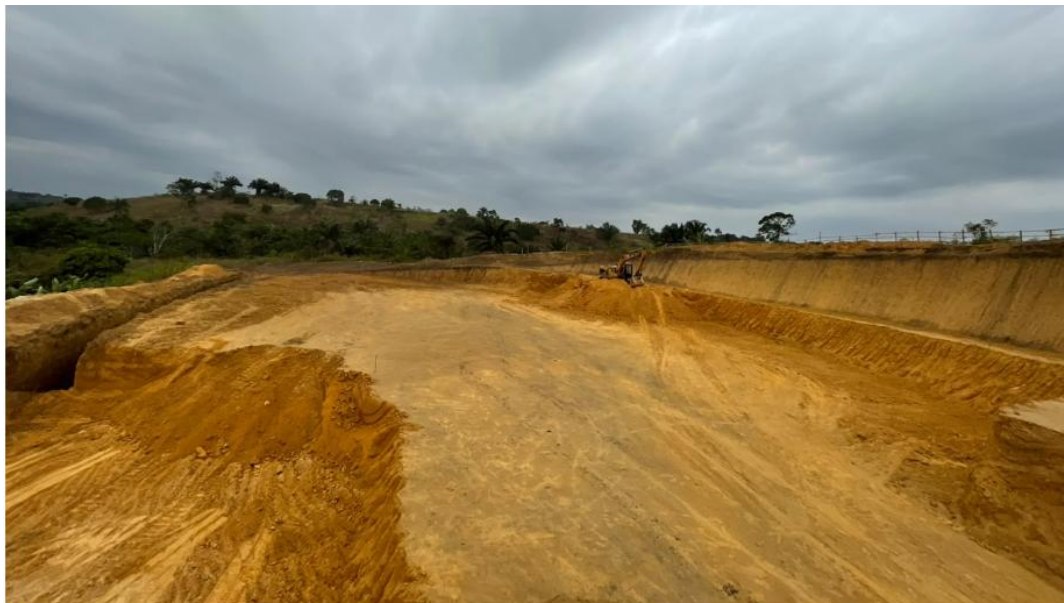
View of the box cut under construction in the Southern section of the orebody
