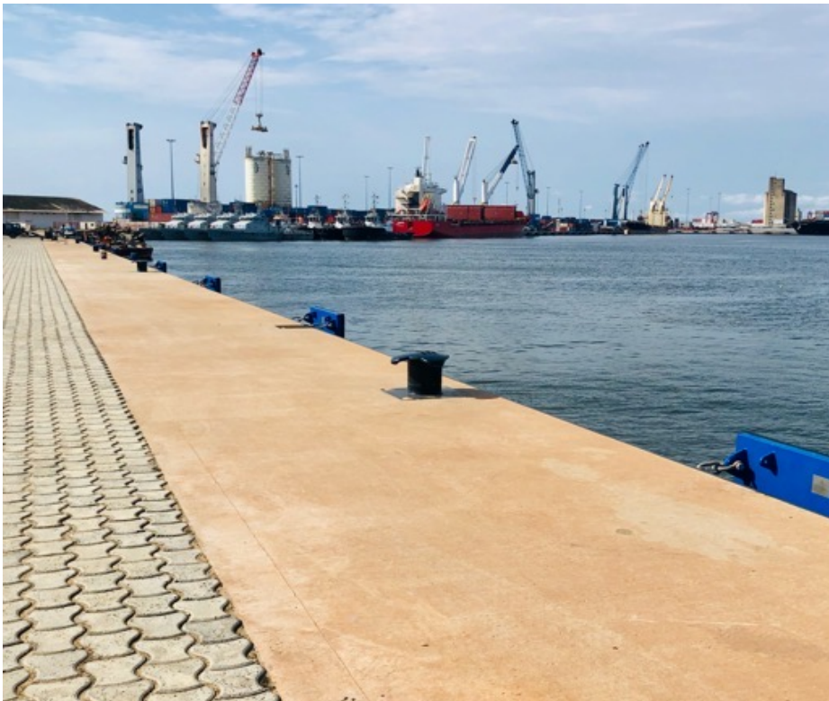
Multipurpose terminal at Port of Pointe-Noire
