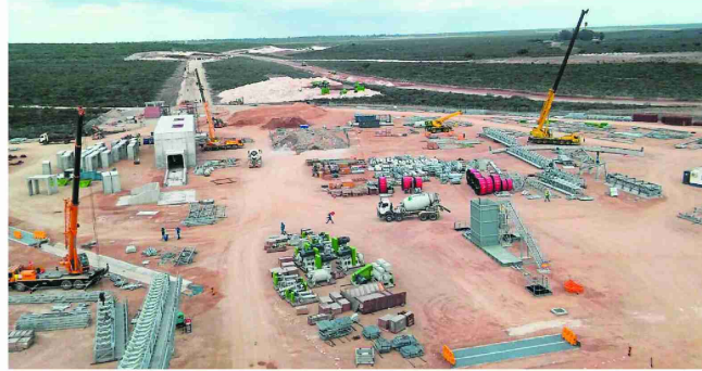
Construction cost on the phosphate mine by September last year had already been around R800 million, but without an integrated water-use licence they can't start mining. Photo: Heléne Meissenheimer
