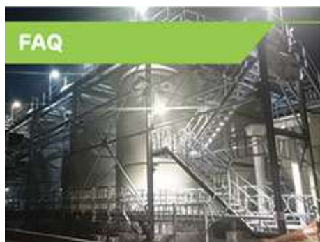
Flotation section of the processing plant at night.
