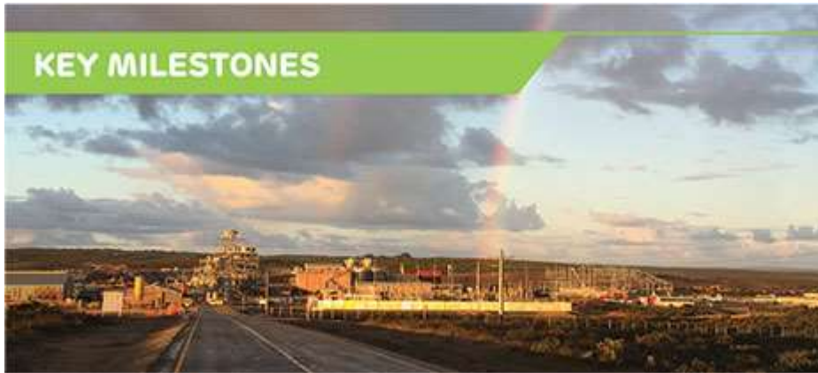
A rainbow over the Elandsfontein phosphate processing plant.
